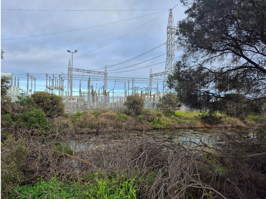
Figure 7: channel of stormwater by Lefevre substation (on east side) 6.8.2026
