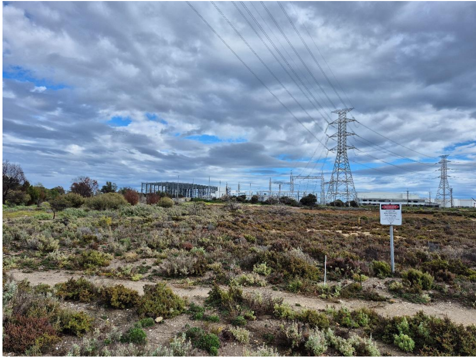
Figure 9: Area south of SEA Gas pipeline, looking west 8.8.2026 – possible lay down area
