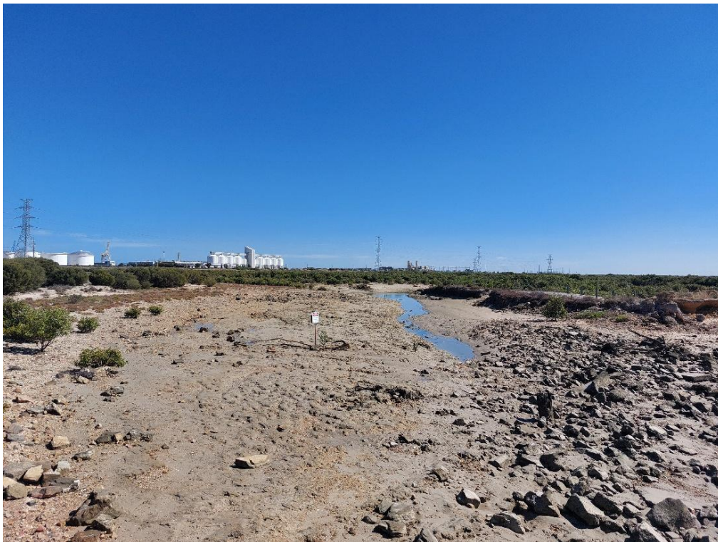
Figure 4: channel into Mutton Cove from major seawall breach 14.3.2026
