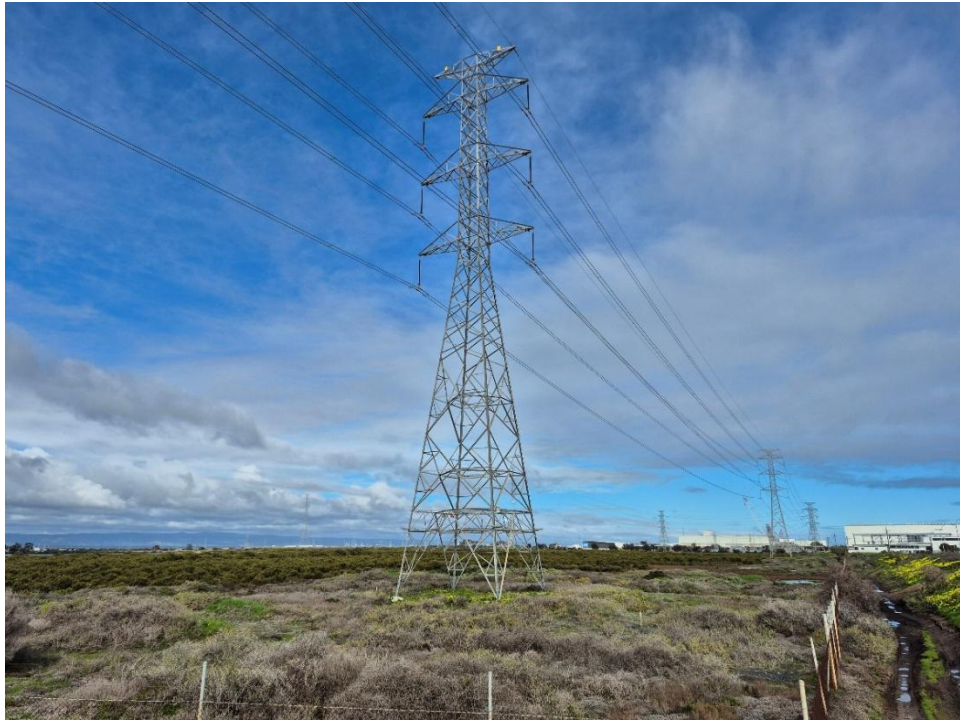
Figure 11: Most northerly transmission tower in Mutton Cove 26.7.2026 - to be removed
