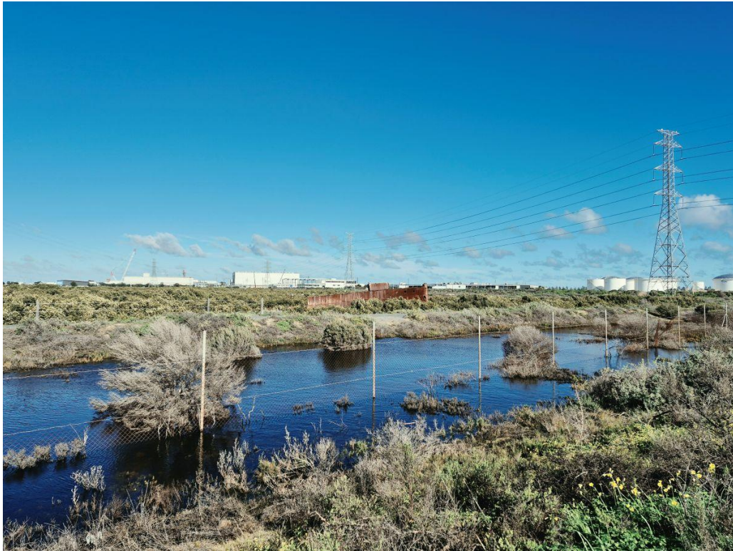
Figure 5: seawater ponding after overtopping northern bank 18.6.2026
