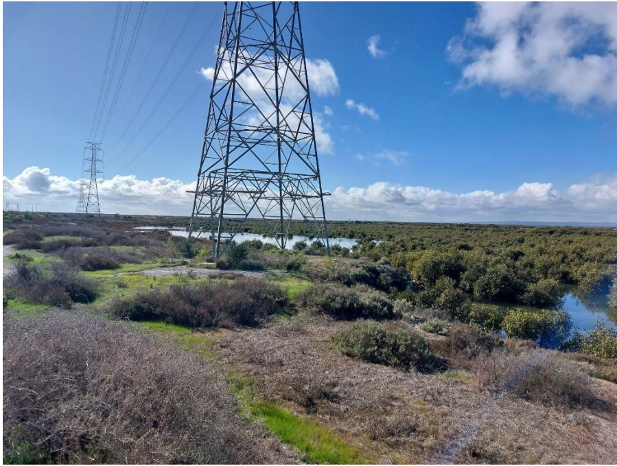
Figure 13: 2nd tower, from north, 6.7.2025 - to be removed
