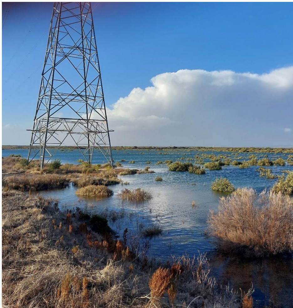
Figure 12: 2nd tower, from north, 26.5.2025 - to be removed
